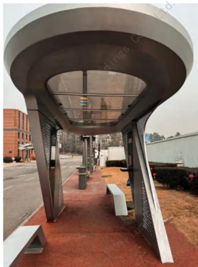
CdTe PV-integrated Storage Station
